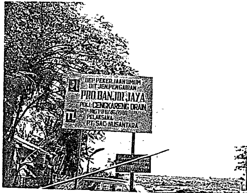
CENGKARENG FLOOD WAY is under construction.
