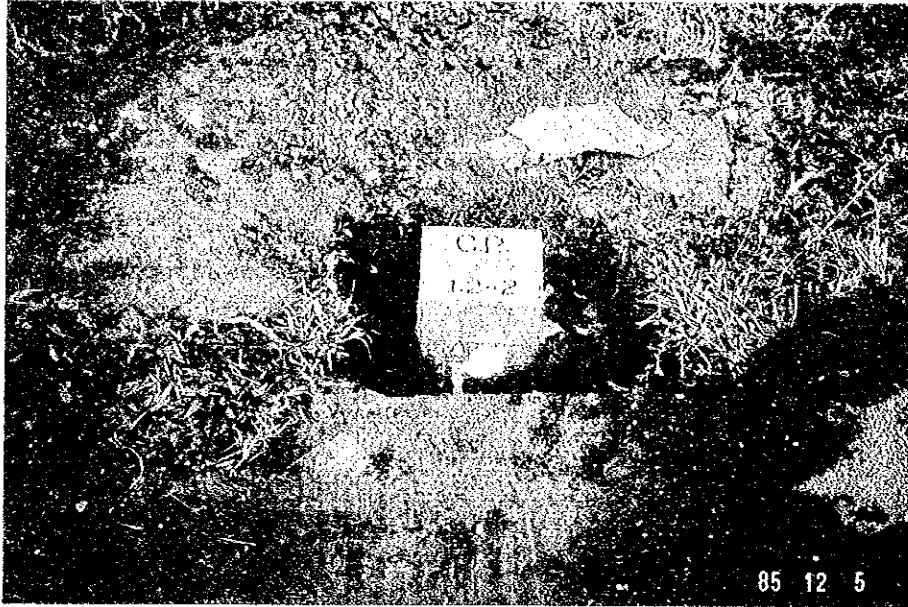
Monitoring point for external deformation of the dam (under installation)
