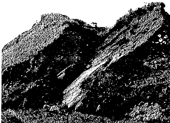
CUT SLOPE SURFACE FAILURE (STRUCTURAL WEAKNESS) C-S.F (S)
