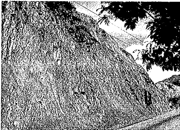
CUT SLOPE SURFACE FAILURE (WEATHERING) C-S.F (W)
