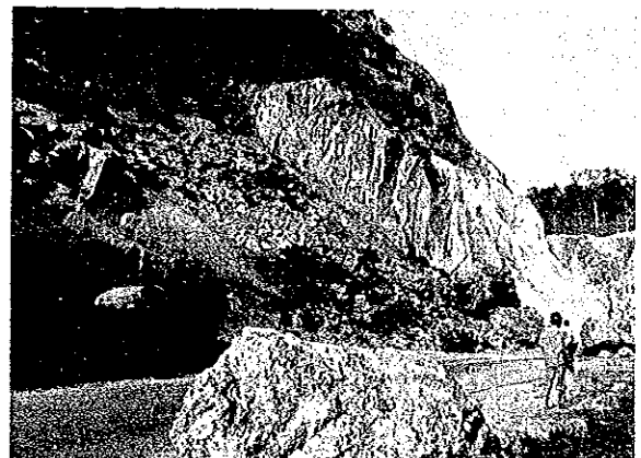
CUT SLOPE DEEP FAILURE (ROTATIONAL) C-D.F (R)
