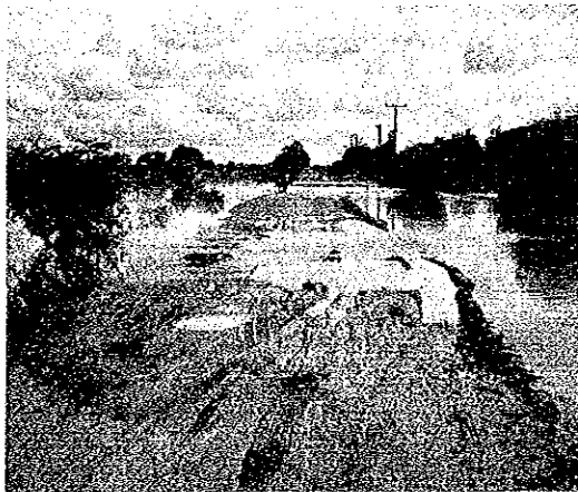
IM-9: Flooding during rainy season
