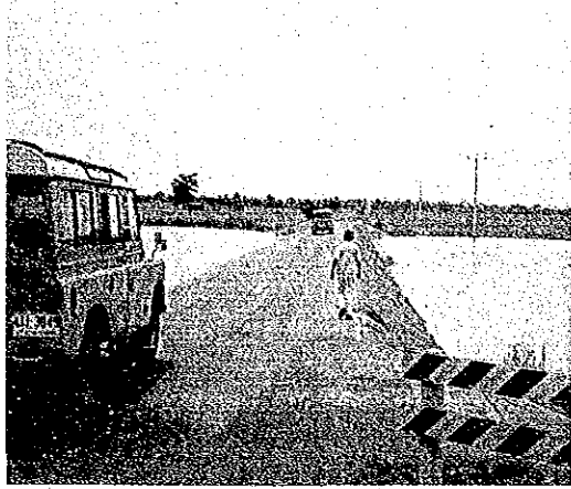
IM-31: Concrete weir
