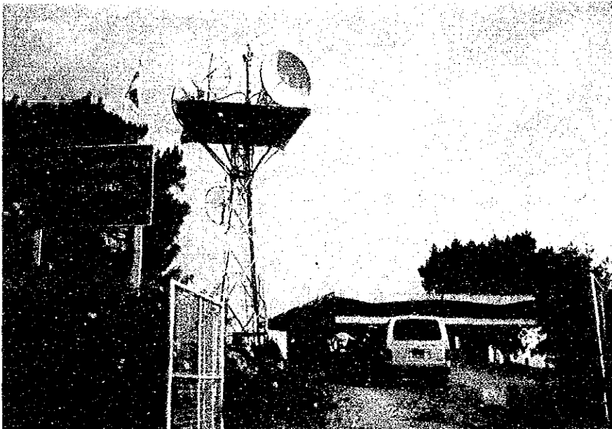
Khao Than Pho Repeater Station ( S2 ) ( TOT, EGAT )
