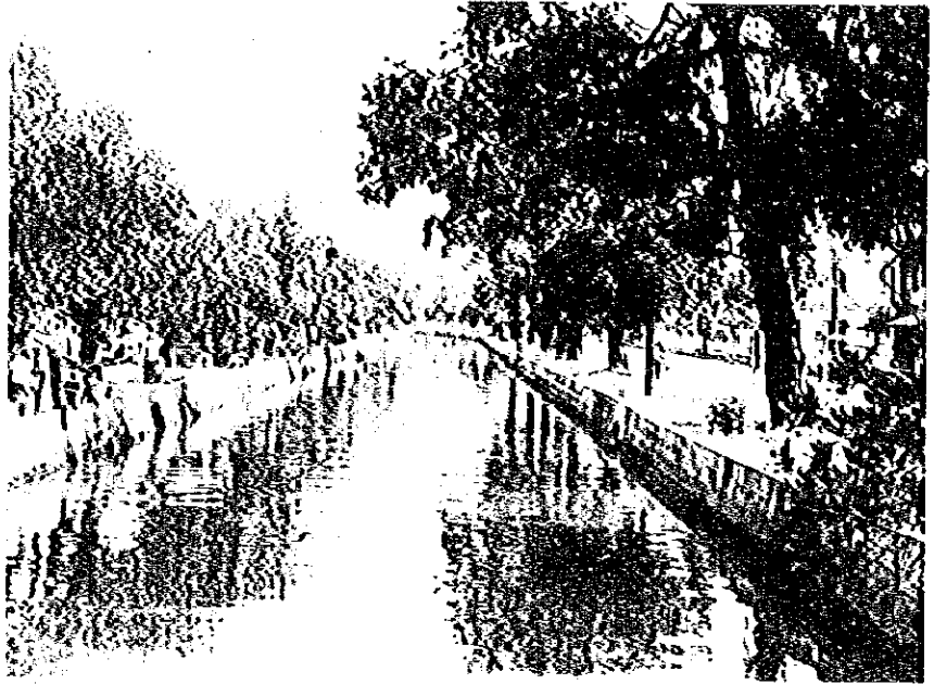
Photo 1 Good Condition of Klong
