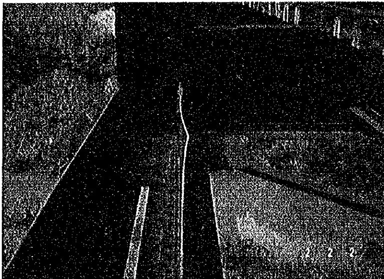
Photo 13 Deformation of Lower Chord
