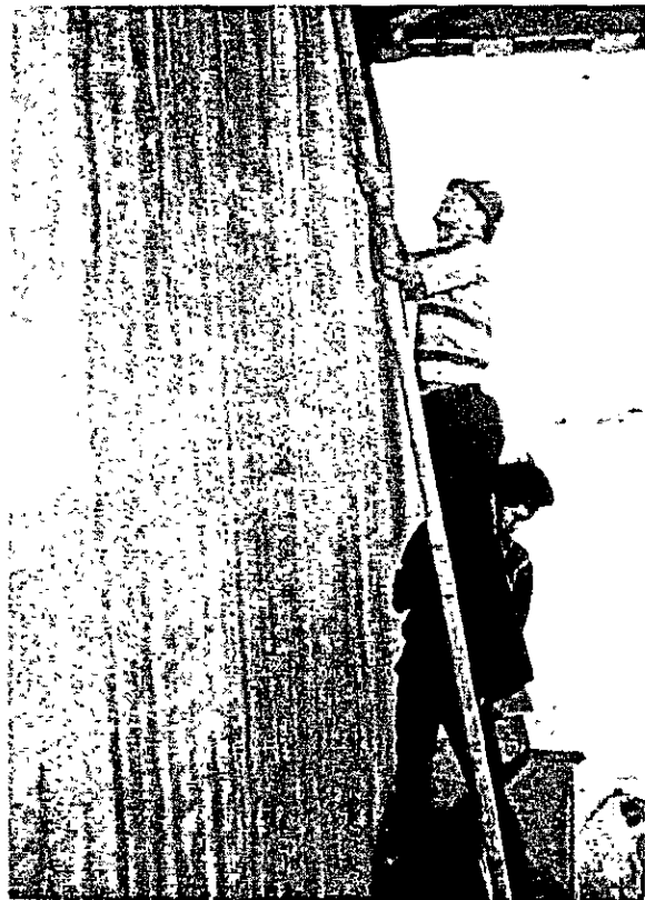
Photo 3-9.4 Visual Investigation at the Pier
