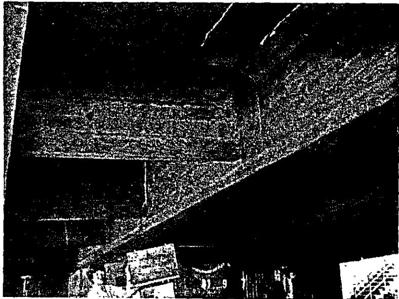
Photo 3-8.2 PC Composite Girder (Thonburi Side)
