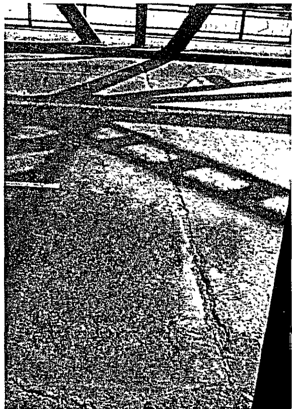
Photo 3-1.4 Pavement on the Carriageway
