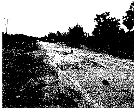
RH-27: Patching and cracks on DBST pavement
