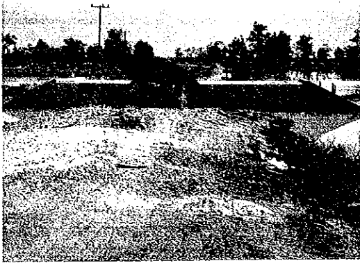
IM-29: Culvert-box under construction
