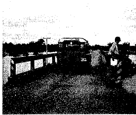
IM-19: Concrete bridge
