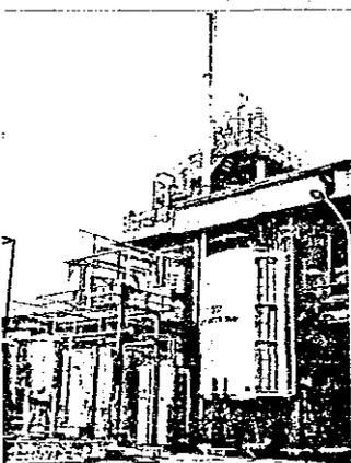
The first alcohol pilot plant from agricultural produce as alternative source of energy is an achievement of the cooperative project between TISTR and the Japanese Association of Industrial Fermentation. The application of innovative technology and sophisticated equipment facilitates energy saving process with the production of 99.5 v/v % ethanol suitable as gasoline substitute for automotive use.
