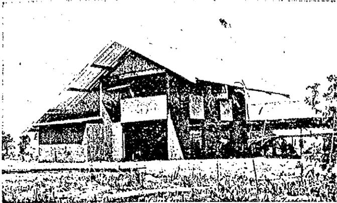
Soil-cement blocks for low-cost rural housing construction.
