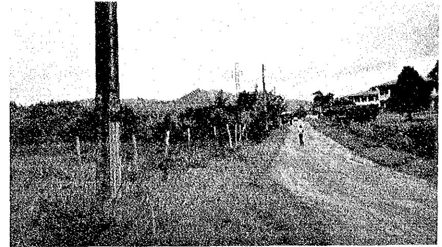
33KV power line crossing the site
