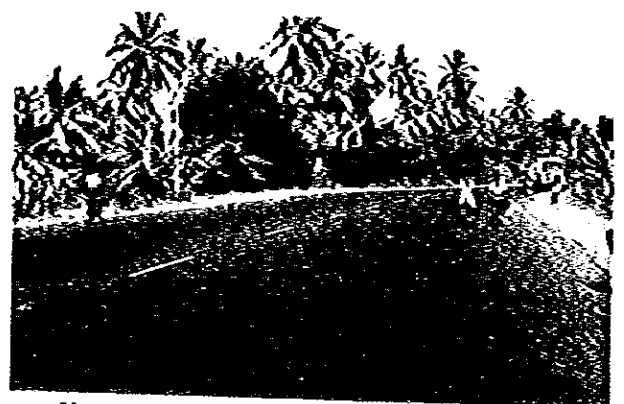
Kandy Road (Near the connecting point of Project A and Project B)
