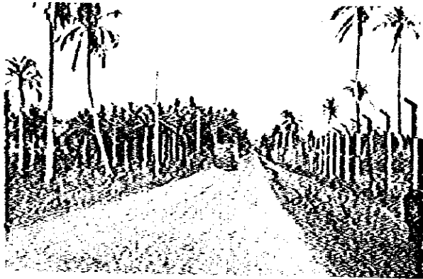
Access Road to Ekala I.C. (On the viewer's side of this road, 1 km long new road is planned for the access to A-3 road.)
