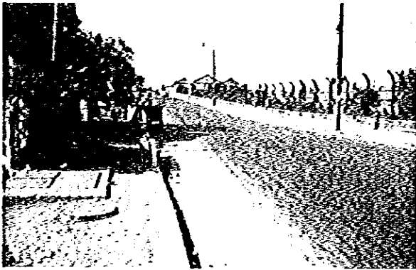
Alutumawatta Road (Near the beginning point of Project B. The New Port Access Road passes through under this road)
