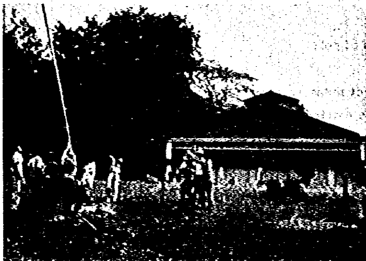
Picture II-4-3 Erection of pole for anemometer
