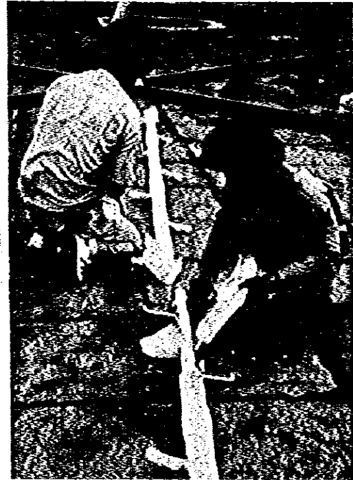
Picture II-1-2-(2) Erection of pole for anemometer
