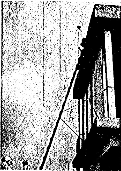
Picture II-1-4-(3) Erection of pole for anemometer
