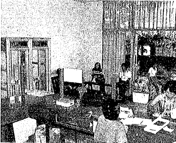
Inter provincial Telephone station of BUTEL (Cabanatuan)
