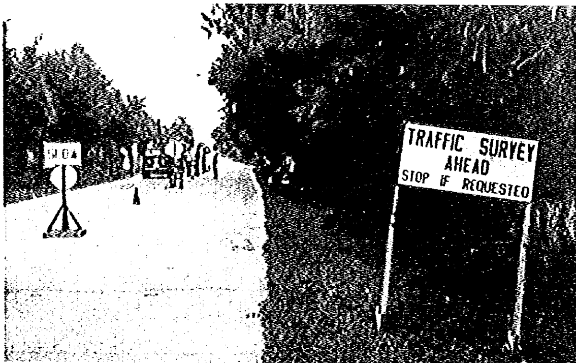
TRAFFIC COUNTING. To determine the total volume of base year traffic and distribution by classification, traffic counting was carried out manually at the same location as the O-D survey on a 24-hour basis with each vehicle type counted separately and by directional flow.
