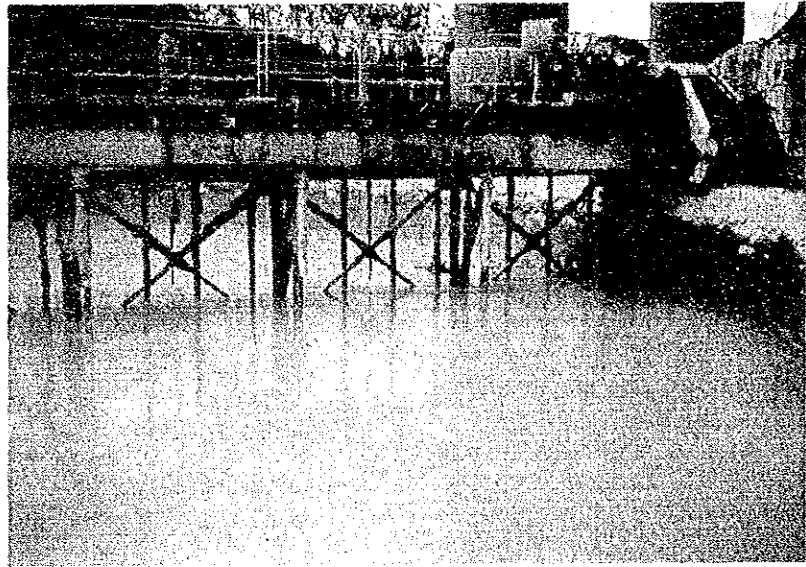
7. Raw material grinding department Slurry basin
