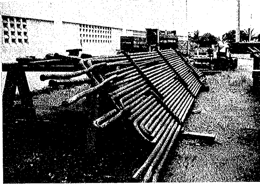
G-2 SECONDARY SUPERHEATER TUBES REMOVED DURING RECENT OVERHAULING
