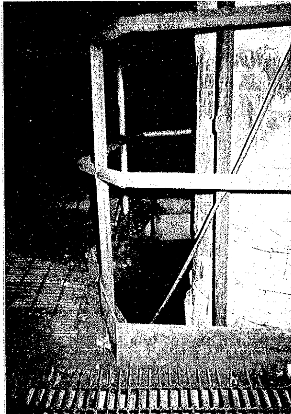
S-1 CRH PIPE & DAMAGED GRATING AT MEZZANINE FLOOR
