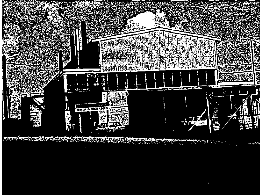
General View of Versailles Power Station
