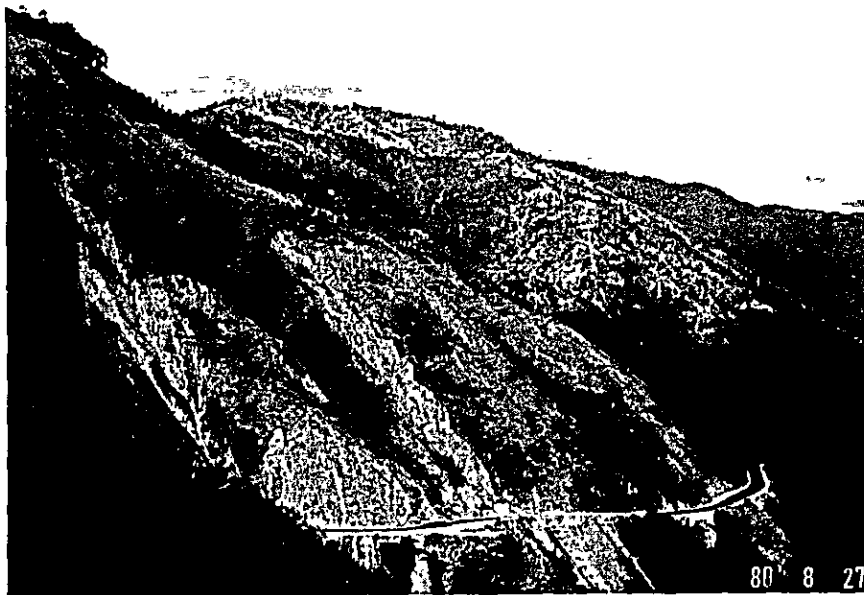
Photo 6-2 The Site in Danger of Landslide
