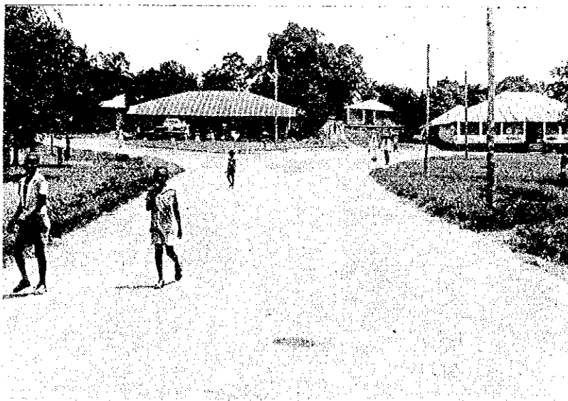
Kamakwie Junction, the project ending point.
