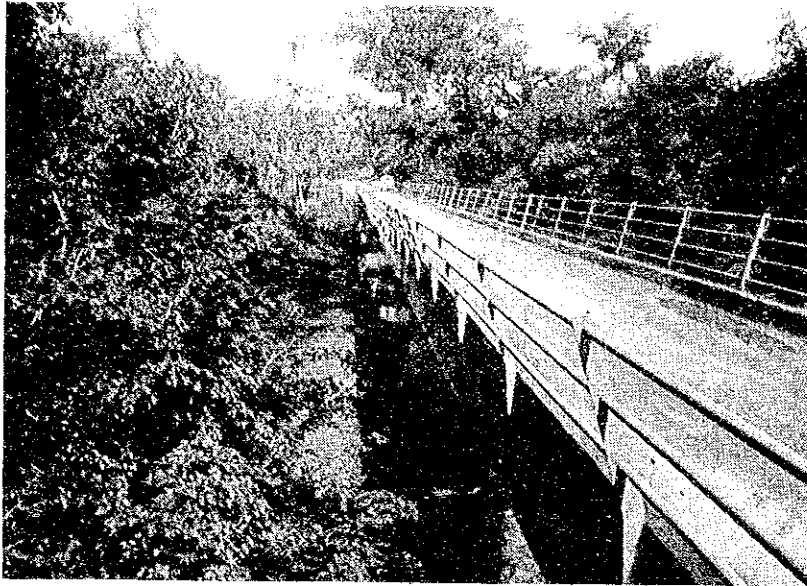
The existing Mabole Bridge.
