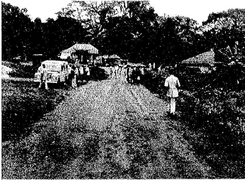
Panlap Junction, where the Project will begin.
