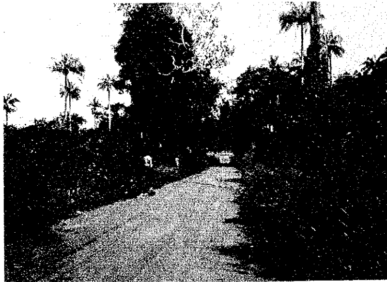
A typical plateau section of the existing road.
