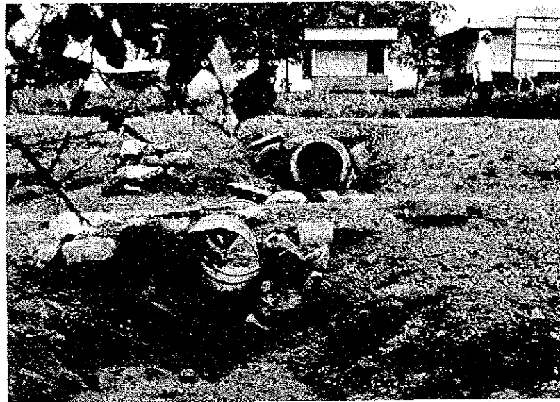
A look at one of the existing pipe culverts.
