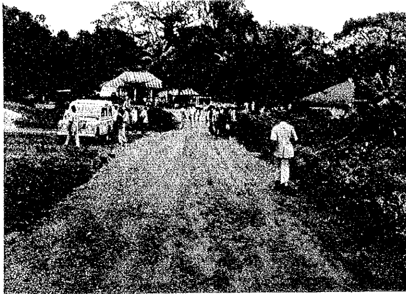
Panlap Junction, where the Project will begin.
