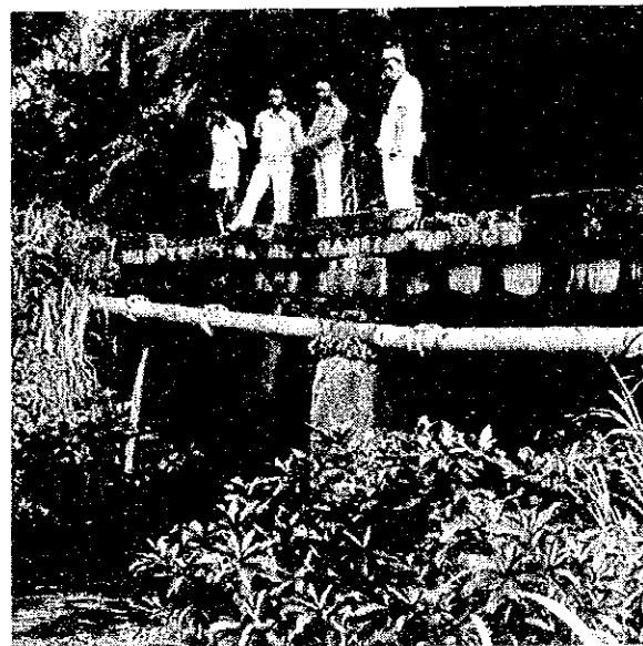
One of the existing I section steel girder bridges.
