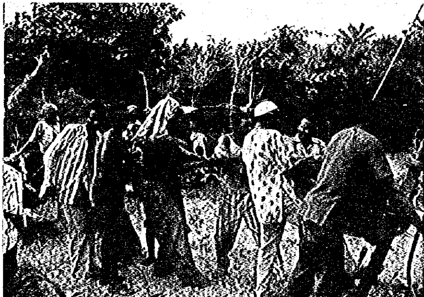
Operation of manual-type boring machine
