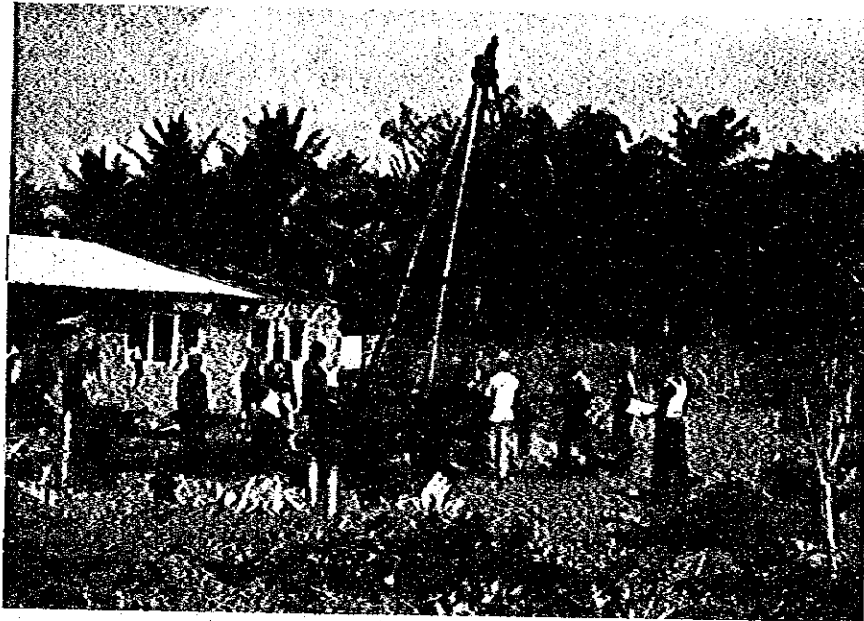
Motor-driven boring machine (1/4)
