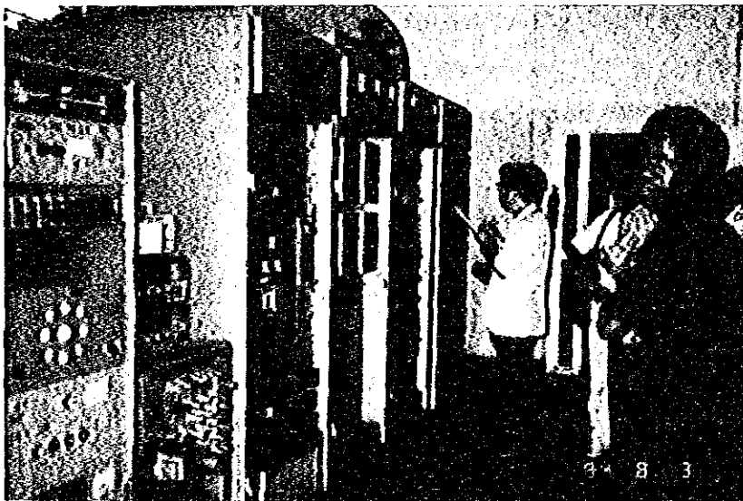
Existing Television Transmitter (Adjangote)
