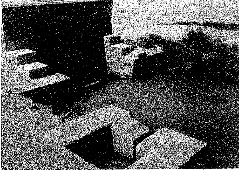
Existing Check and Vent for Intaking Irrigation Water
