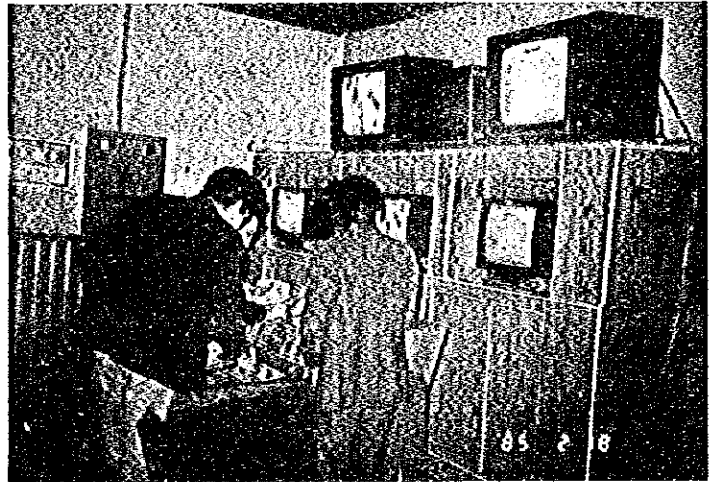
MASTER CONTROL ROOM送出監視卓
