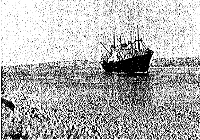
Suez Canal Near T/L Crossing Point
