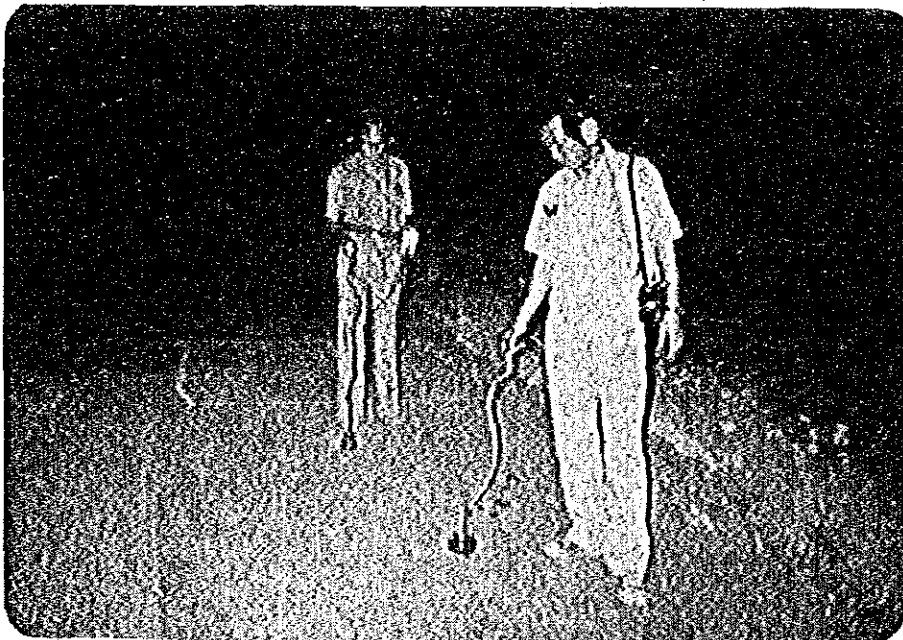
Leak detection at Kafr El-Eshara area of Zagazig city
