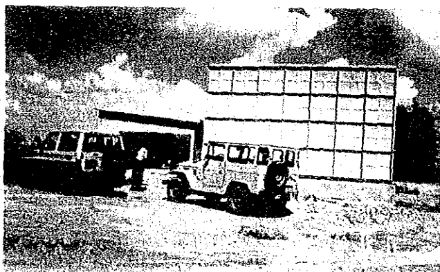
Pump and reservoir tank (1st-Phase Grant, Harad).
