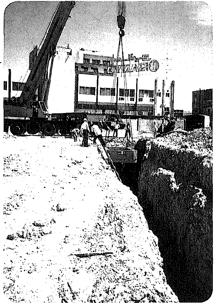
Test trench construction
