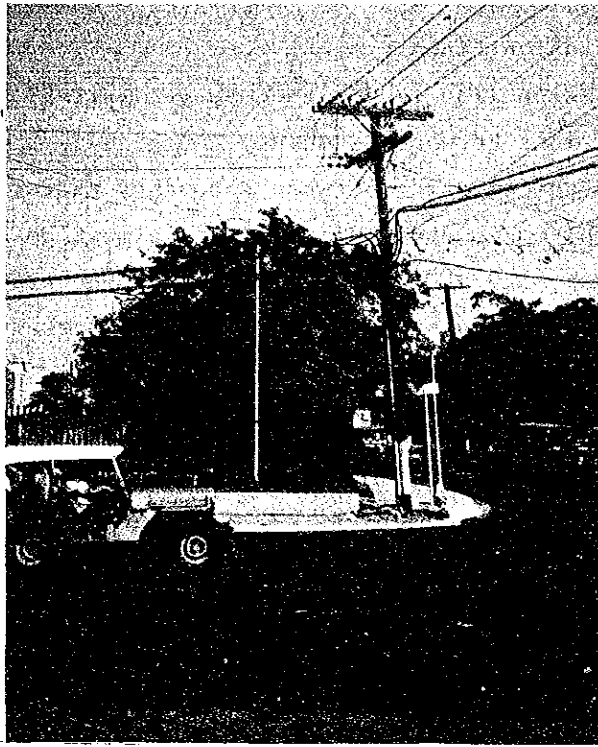
Telephone Cable mounted on a pole (At Manila)
