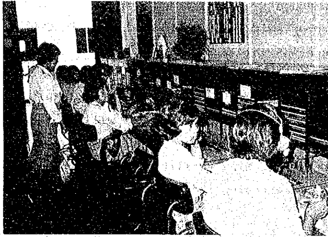
Toll switch board of Manila Toll Exchange Office
