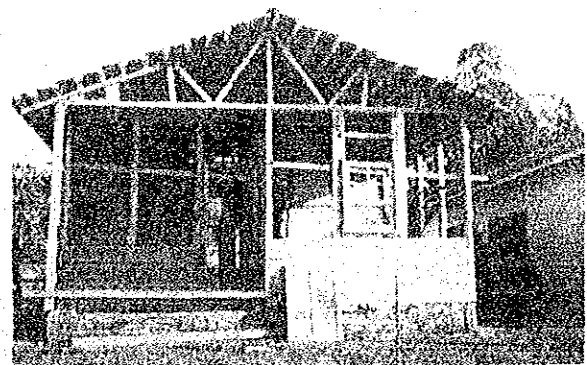
Photo V-8 Prefabricated living house by utilization of small-size logs
