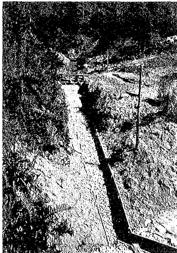
Photo II-12 Execution of simple hillside conservation work (channel)
