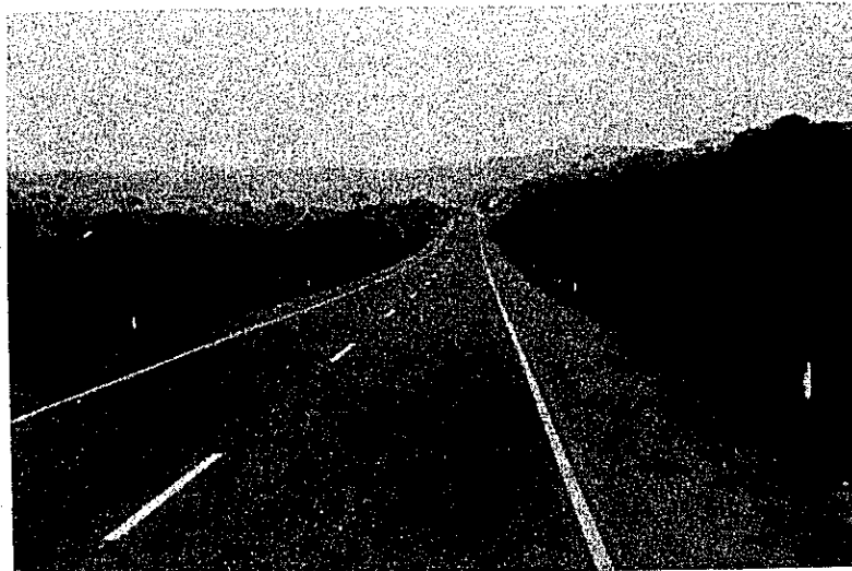
No. 18 Arterial road linking Brazilia and Belo Horizonte.
