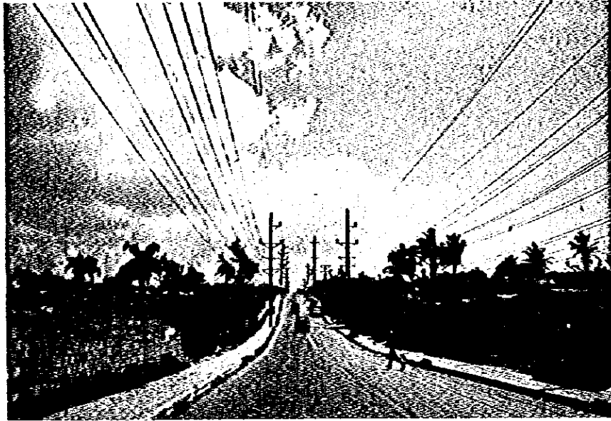
69kV Transmission line (Tangent structure)
