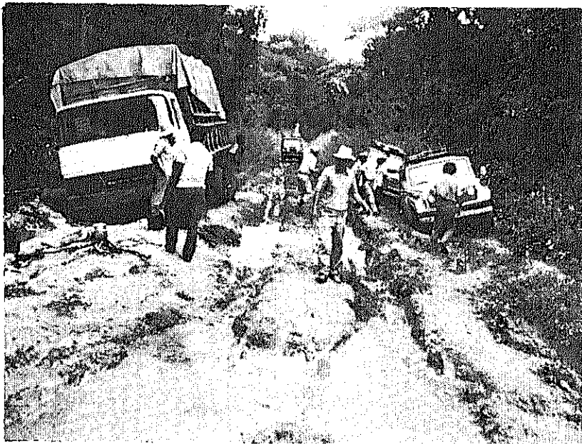
Photo. 2. Road conditions in wet season at PK 78 (between Likati and Bondo)
