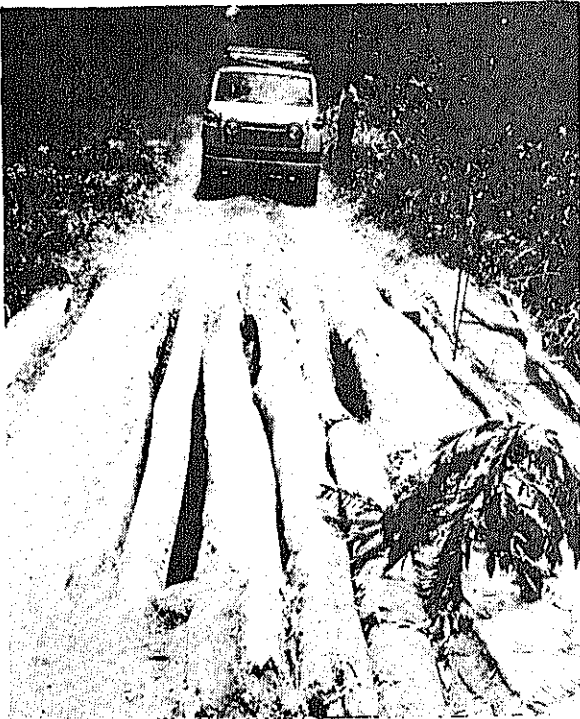
Photo. 7. Wooden bridge at PK 48.7 (between Dulia and Likati)
