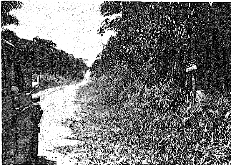
Photo. 1. Road conditions in dry season at PK 101 (between Kisangani and Banalia)
