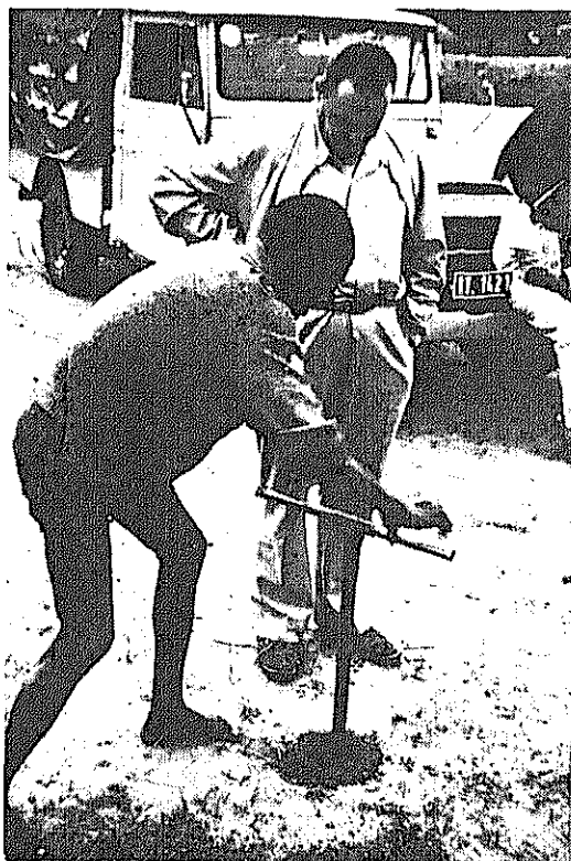
PHOTO 15 Auger Boring at PK 45 (between Buta and Dulia)
