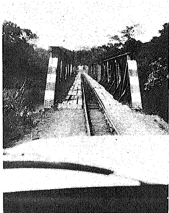
Photo. 8. Libogo Bridge commonly used by railway and road at PK 77 (between Likati and Bondo)
