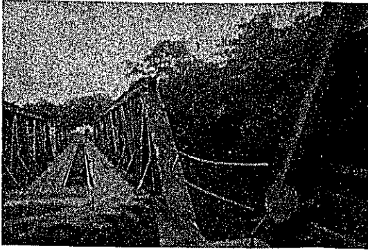
Bridge with road and railway 鉄道との併用橋
