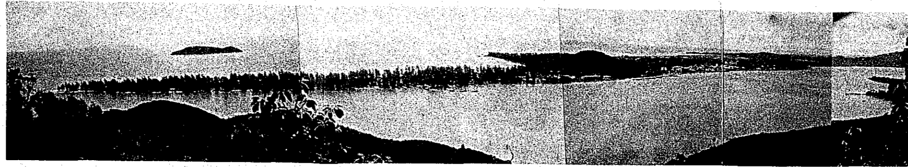
Photo-1 Perspective View of Songkhla Port and Surrounding Area
