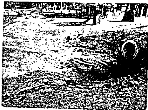
Current Sewage Discharging Pattern
