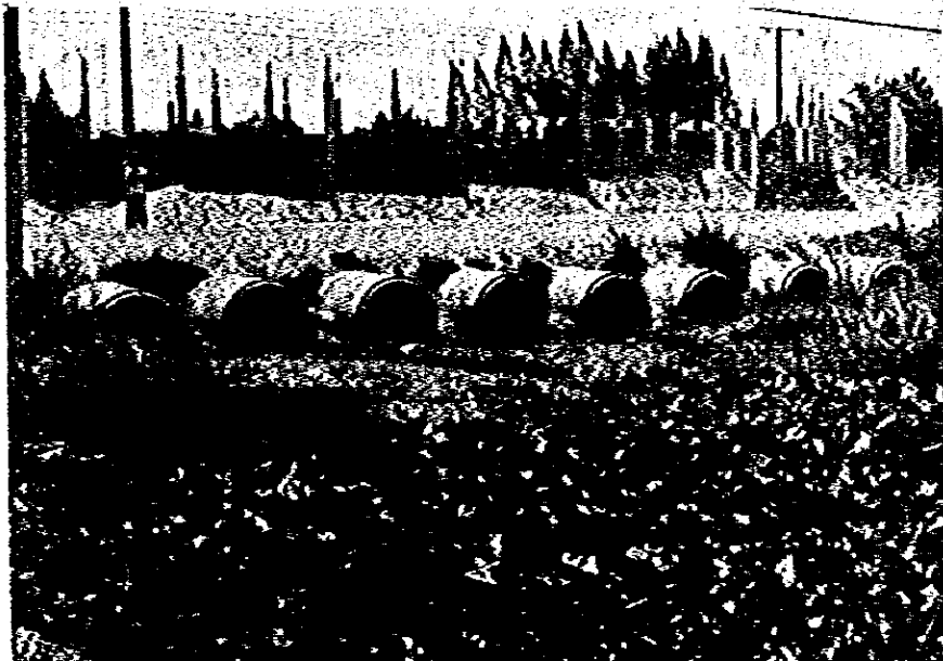
Existing Pipe Culverts (Central Pattaya Area)
