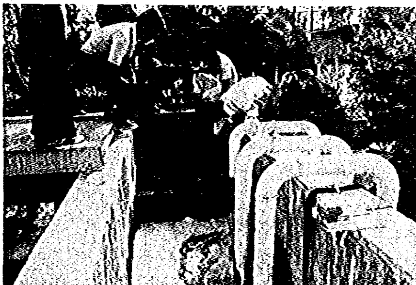
Wastewater Quality Survey at a Hotel in Pattaya
