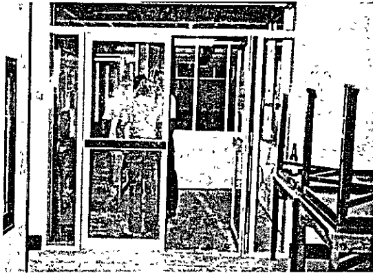
Entrance of Information Processing Institute in Thammasat University (under construction)
