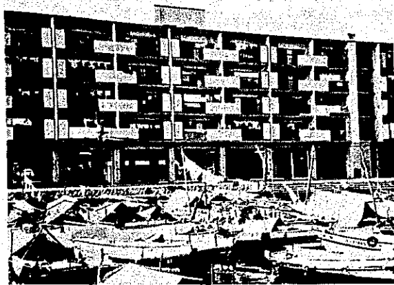
An apartment house for fishermen in the City of Onomichi, Hiroshima Prefecture. The first story of the house is used as fish landing places and offices of the Fishermen's Cooperative Association.
