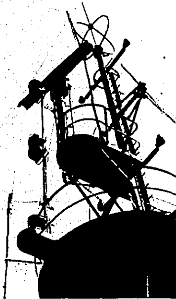
NNSS antenna on the main mast
