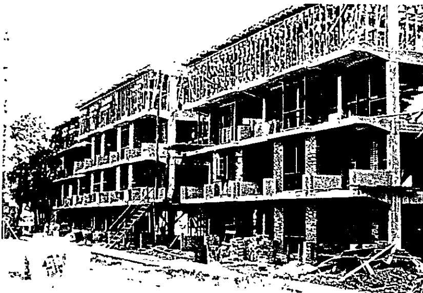
Photograph 2.3.5 U Wisara Housing Project
