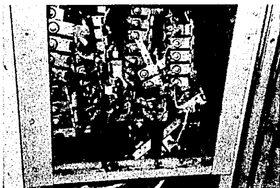
Part of the damaged medium wave transmitter (10 kw)
