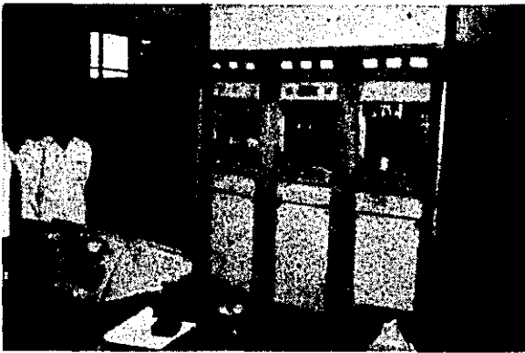
Medium wave transmitter of Chittagong Station (10 kw)
